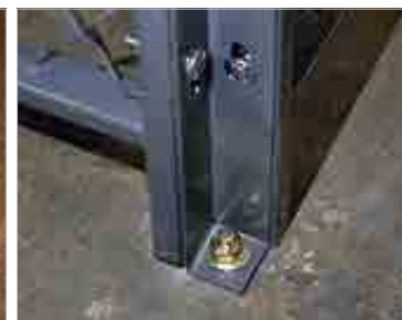
Corner post mounts flush with wall line to eliminate trip hazard
