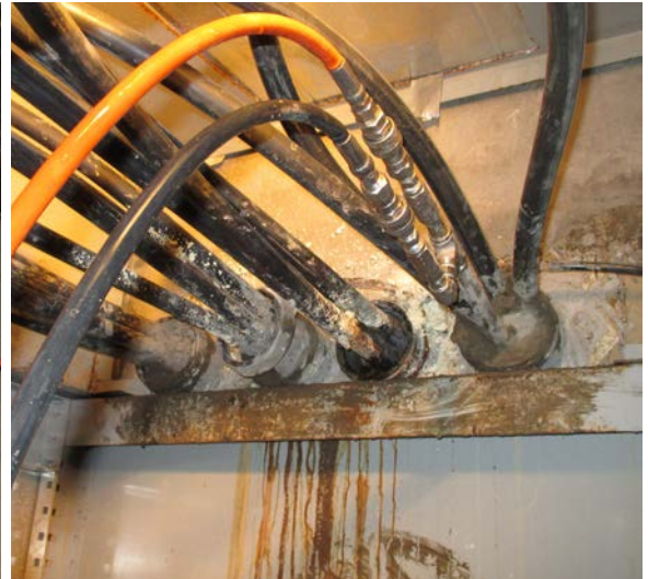
CONDUIT SLEEVE TO CABLE(S) PENETRATION (ANNULAR INJECTION)
