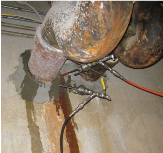
CORE TO PIPE PENETRATION
